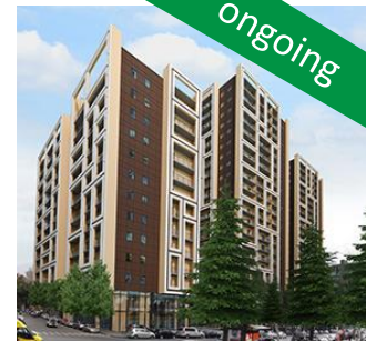
Apartment building: Kazbegi avenue II Completion status: 7% Construction start date: Jun 16
