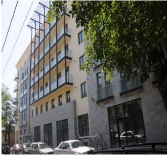
Apartment building: Chubinashvili street Completion status: 100%
