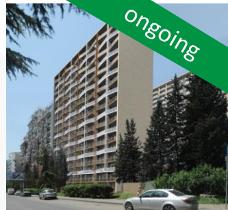
Apartment building: Kartozia Street Completion status: 21% Construction start date: Nov 15
